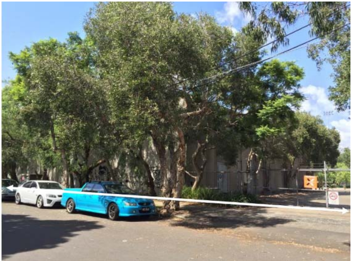
Figure 4: Site viewed from Huntley Street
