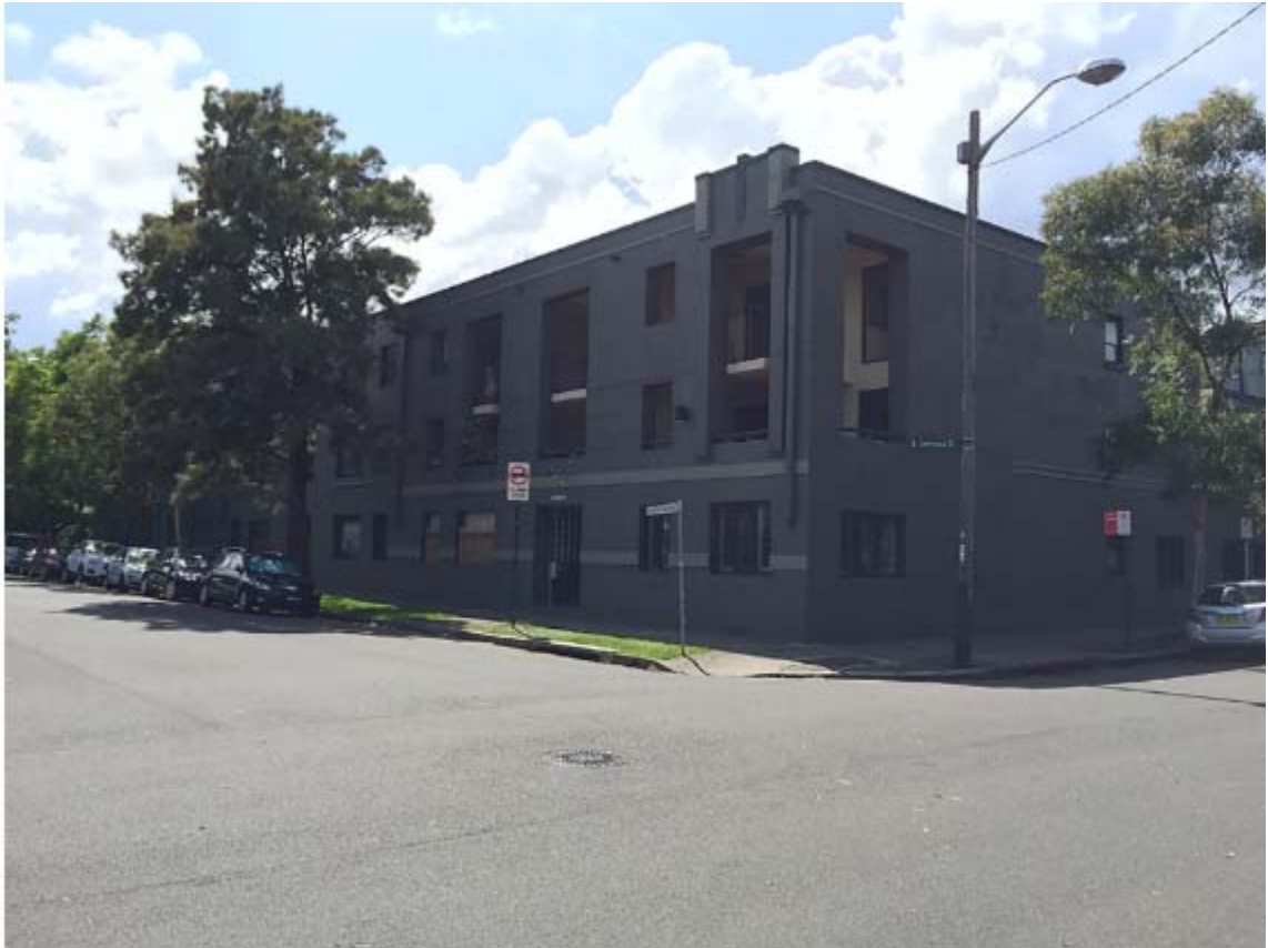
Figure 5: 288-302 Lawrence Street to the north of the site
