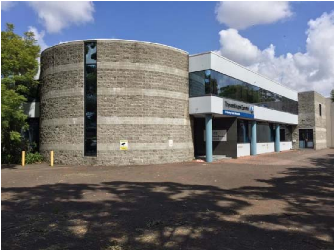
Figure 8: Existing two storey development located on the site
